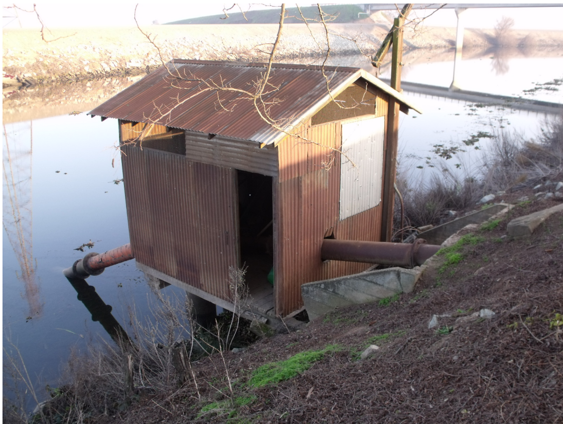
Photo 6. Pumphouse previously found in the same location, since removed. (USACE inspection photo, 2015.)
