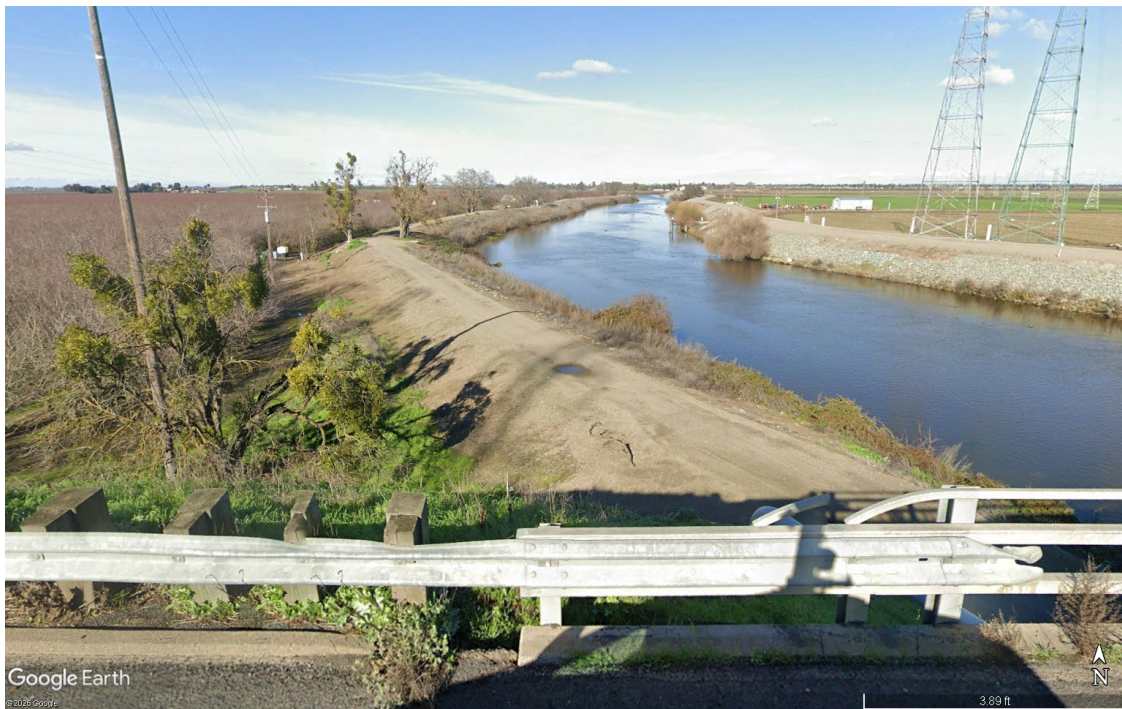
Photo 5. View of levee and pump looking south from Howard Road. (Google Earth, 2026)
