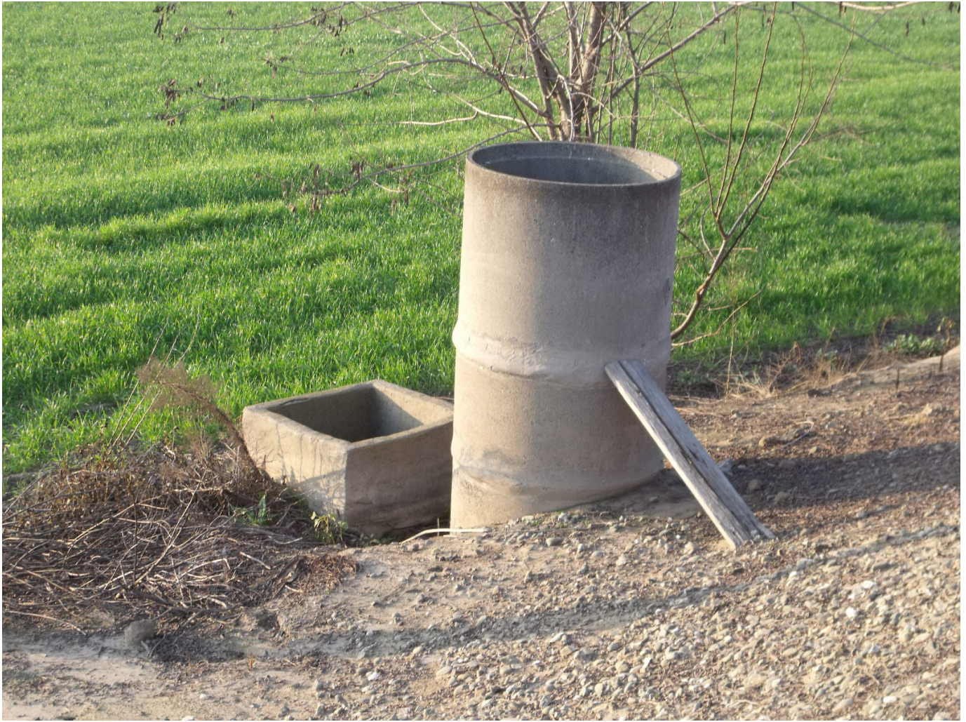
Photo 7. Riser pipe and box originally located on the landside levee hinge, now removed. (USACE inspection photo, 2015.)
